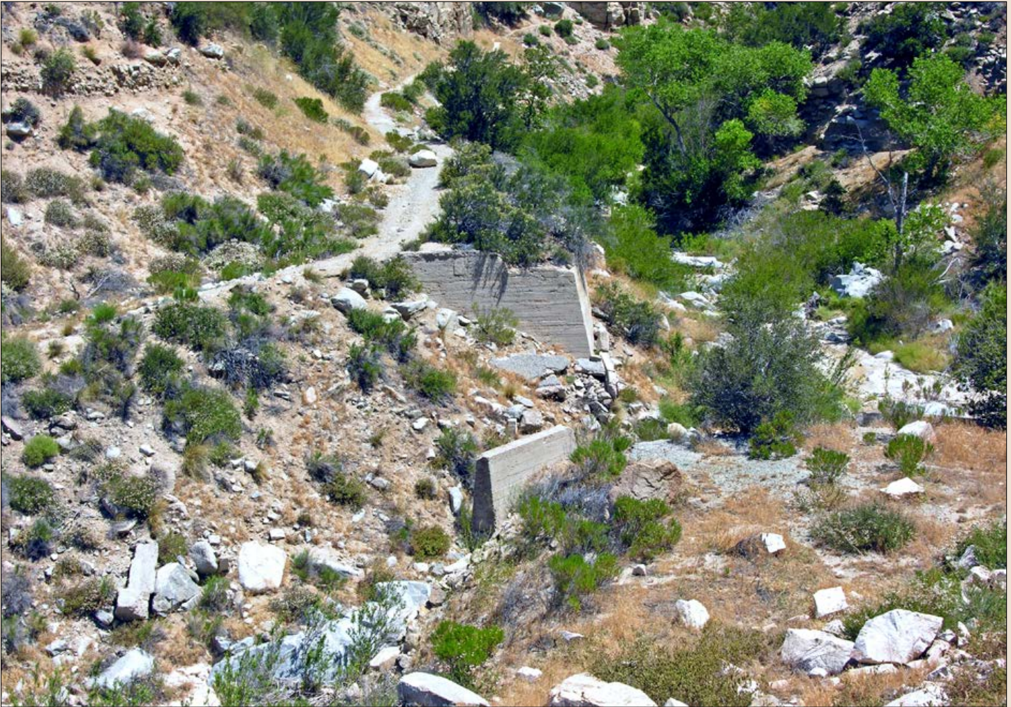
Old bridge abutment in Crowder Canyon
