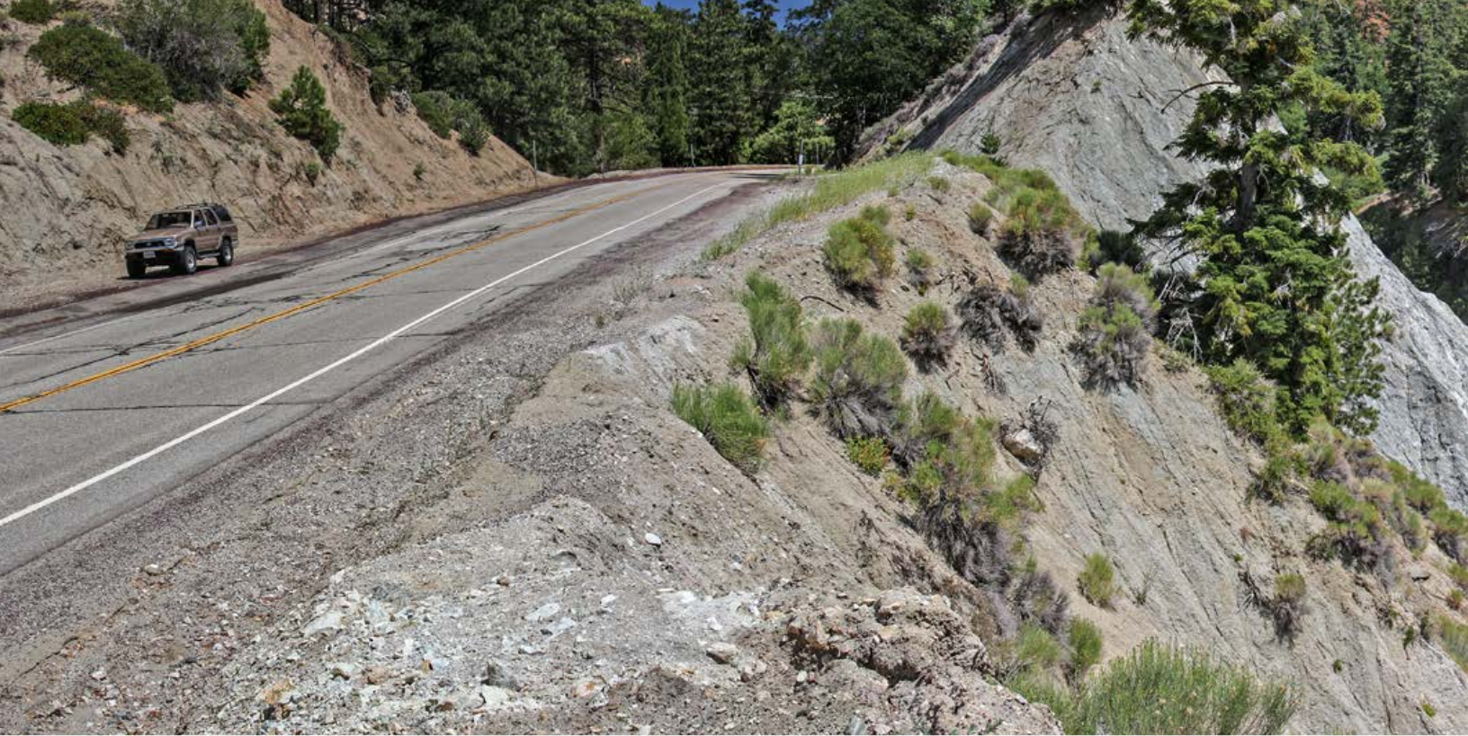
Deep gorge formed by the fault along Big Pines Hwy
